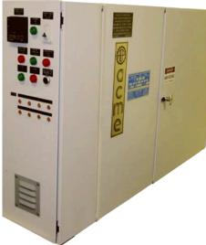
The integral Bi-Energy control option will allow the operation of both the new electric boiler(s) and the existing oil or gas-fired boiler(s) according to outdoor temperature or special requirements.
